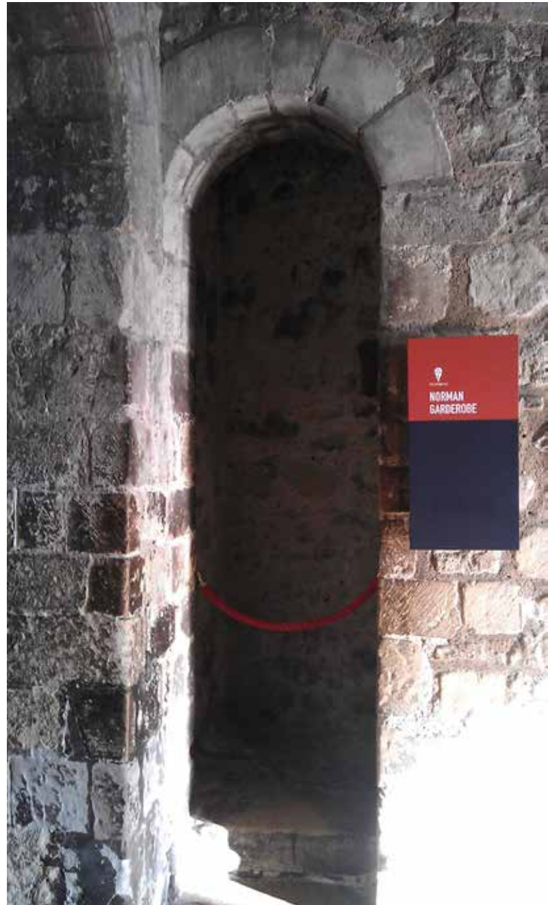
One of the six original Norman Garderobes found throughout the White Tower. This one is located on the First Floor.
