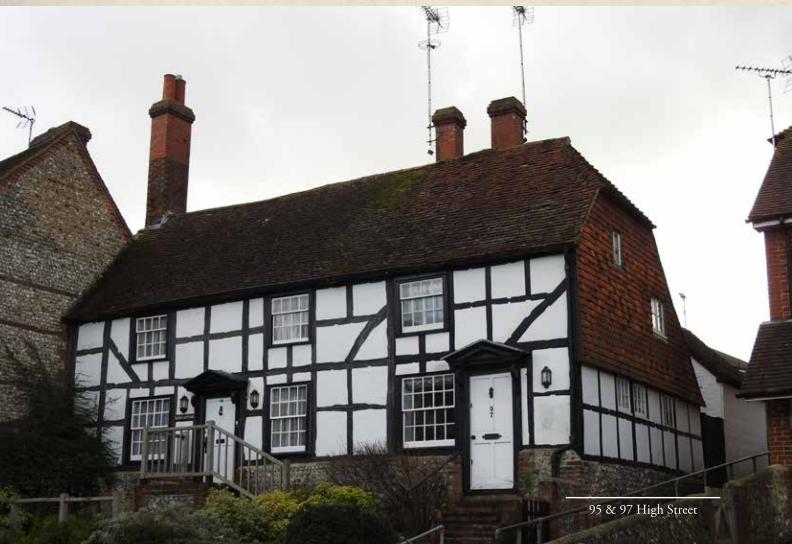
Old Workhouse Cottages
