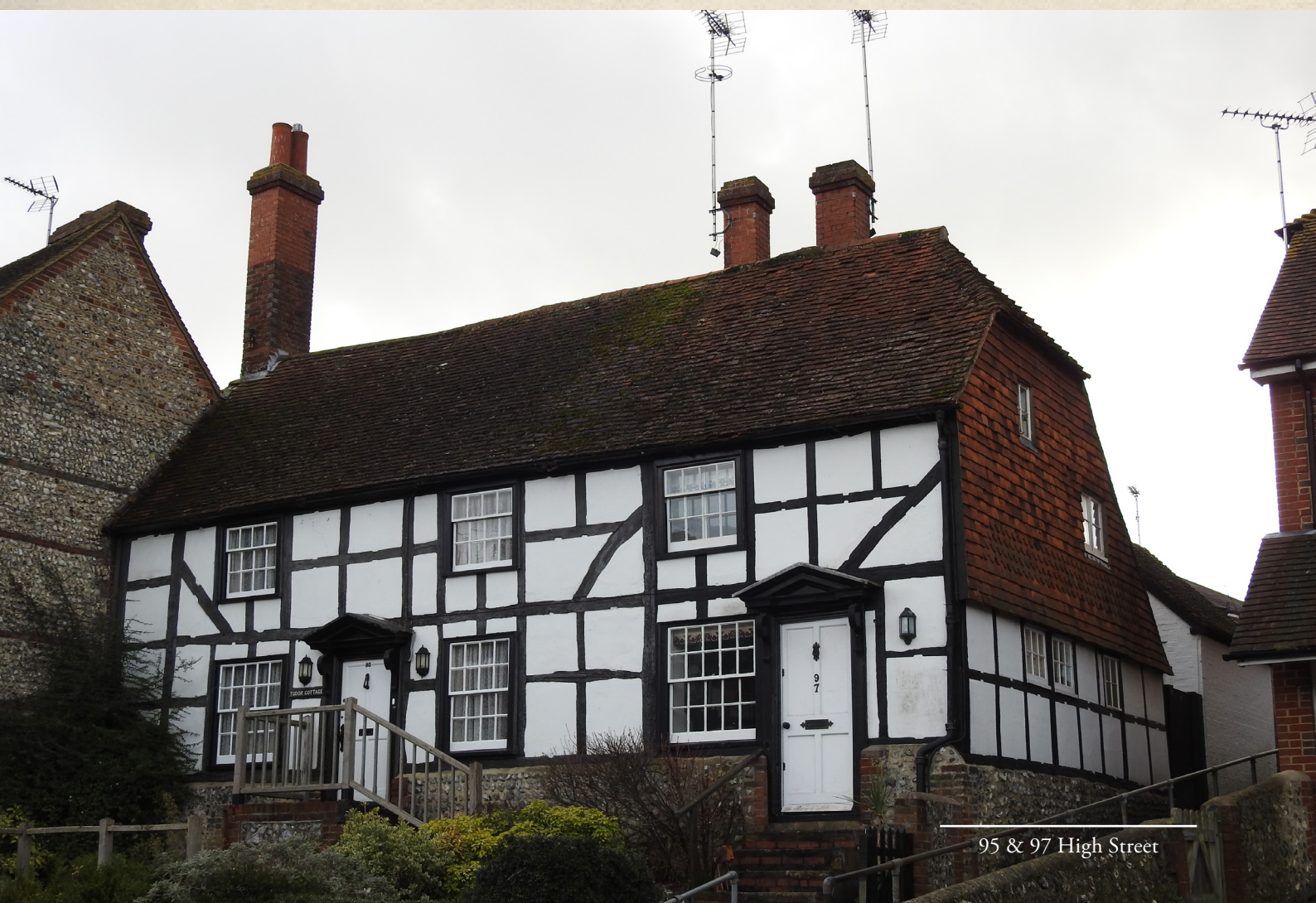
Old Workhouse Cottages
