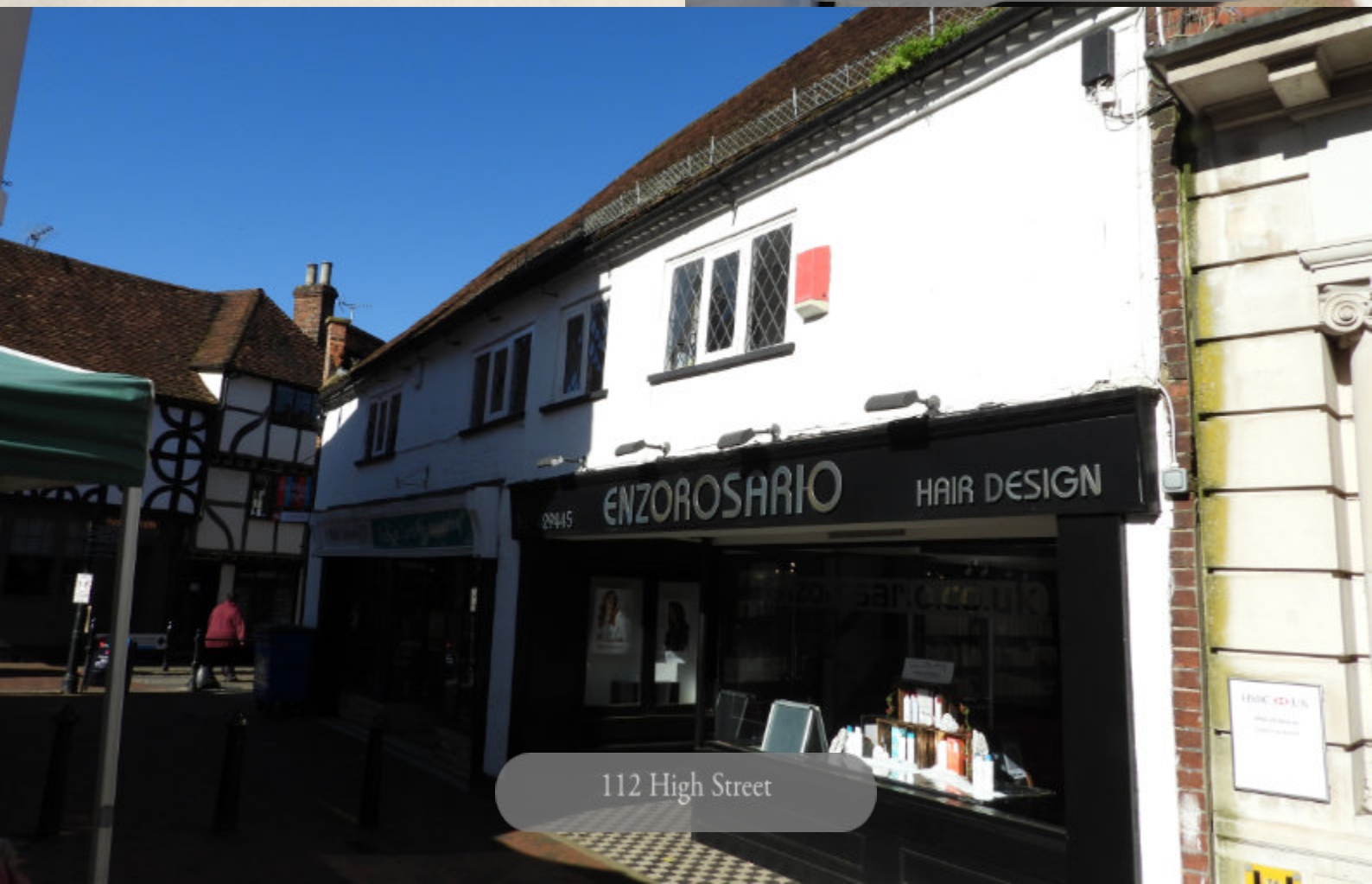
The last remaining visible timbers of 107-109 High Street
